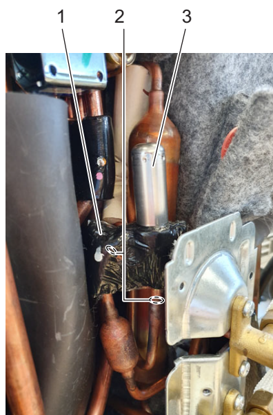
Figure 3-20: Removing the expansion valve
